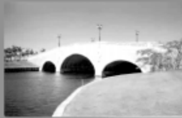
Concrete Arch Bridges
